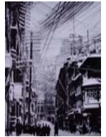
New York Telephone Cabling, 1888
