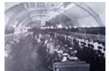
Telephone Central Office in London, 1926
